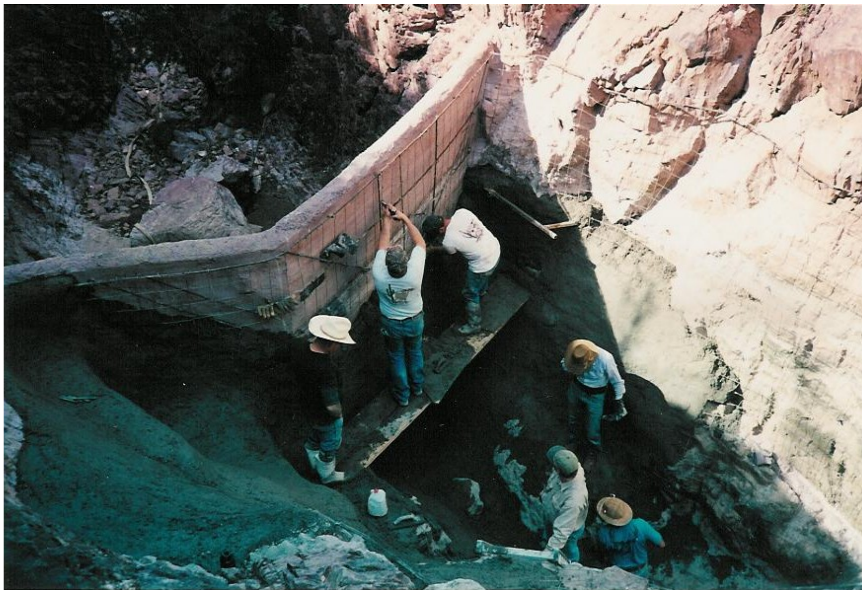
Signal Peak Pothole, Gila Bend Mountains. Tank is being sealed with a mortar lining.
